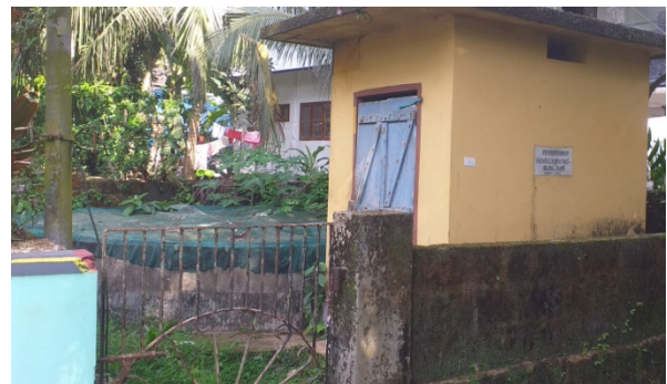
Affected well for water supply
