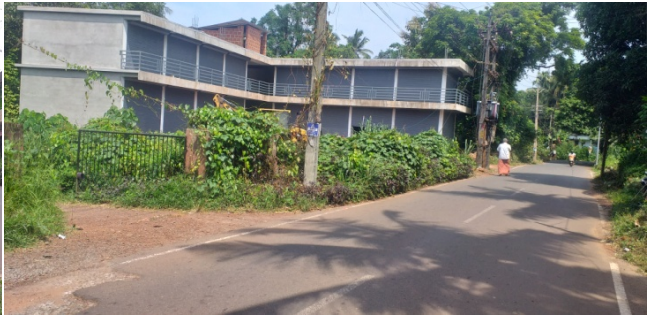
Affected property:- for bus bay
