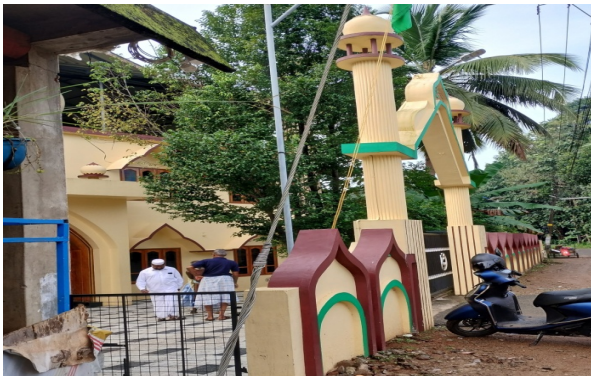
Affected Masjid wall & Khabarsthan
