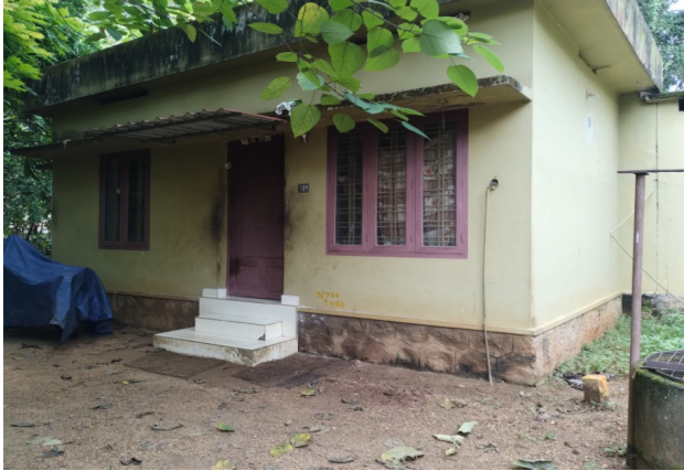
Affected frontage of the House
